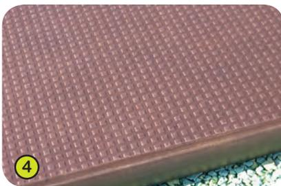
4- **The platform floors** are made from a 12.5mm thick, textured, non-slip compact material (HPL).
